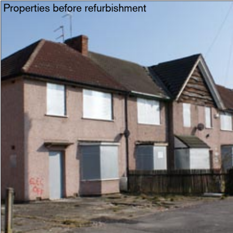
Properties before refurbishment
